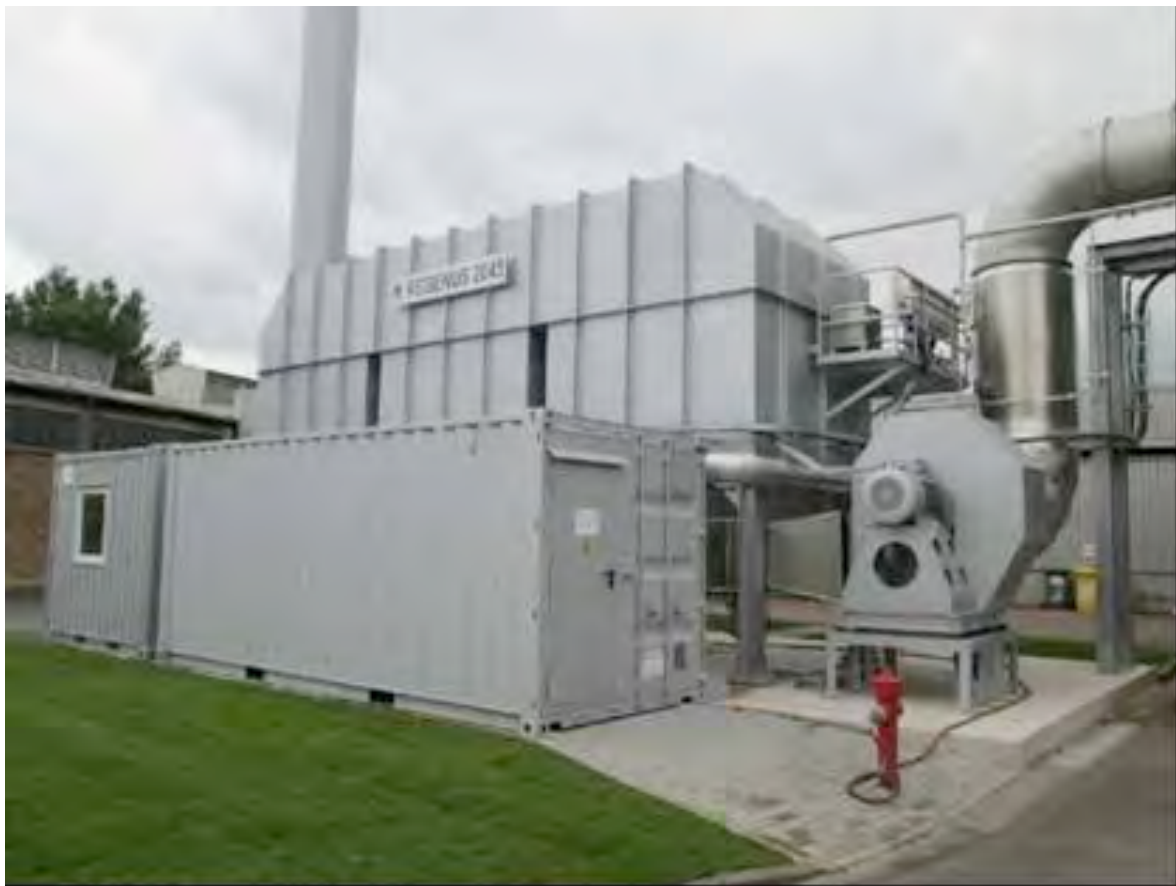
Figure 7: Picture of the waste air treatment unit with control room, enclosure of the plasma unit and air blower
